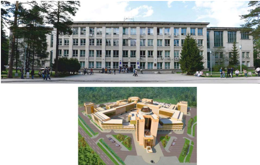
Fig. 18. Novosibirsk state university: the current main building ( top ) and a new main part of NSU under construction ( bottom ). Source: http://www.nsu.ru .
